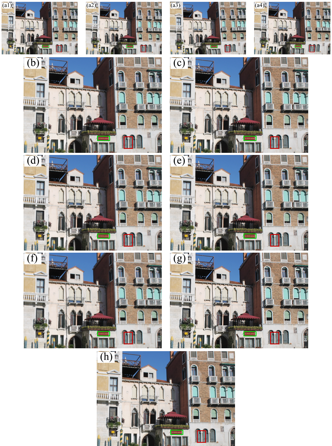
Figure S3. Real example: Building 2 .
